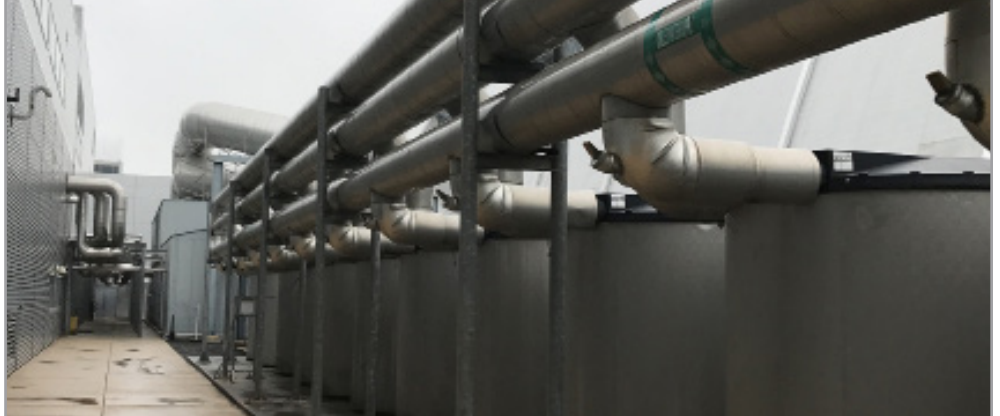
The newly upgraded ice farm on top of the Steven F. Udvar-Hazy Center.
