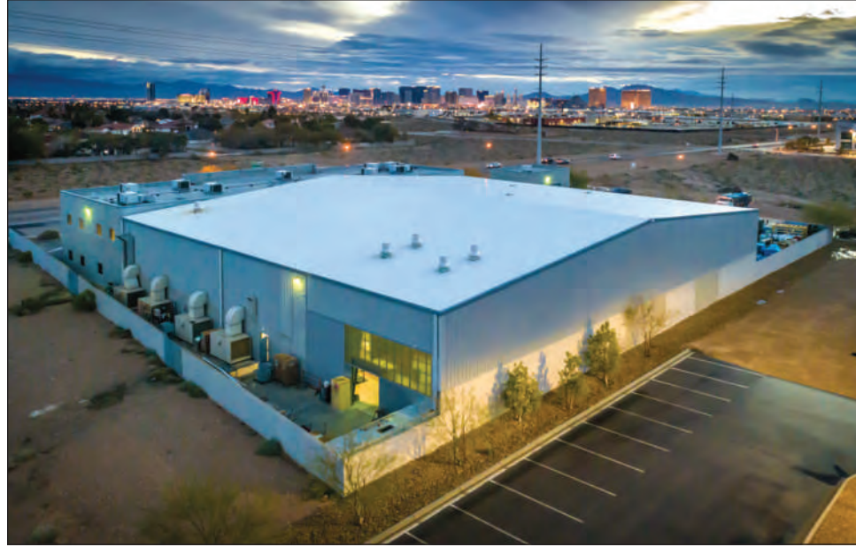
Harris' Las Vegas office and prefabrication Facility.
